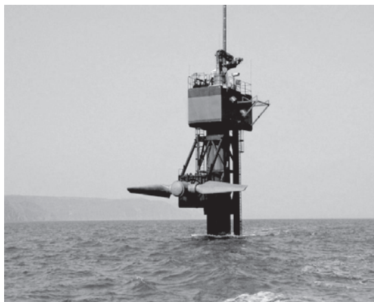
Seaflow tidal generator. Here the turbine assembly is raised for maintenance. It will slide down the pile and operate underwater for electricity generation
